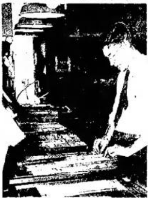
FINAL CHECK-UP BEFORE LOCK UP is being done here by foreman Gene Murphy. Murphy marks the advertising copy for type styles and proportions fit out to the Linotype machines. He also gives the final O.K. on the type page before it goes to the Stereotype department.
