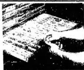
FINAL CHECK-UP BEFORE LOCK UP is being done here by foreman Gene Murphy. Murphy marks the advertising copy for type styles and proportions fit out to the Linotype machines. He also gives the final O.K. on the type page before it goes to the Stereotype department.
